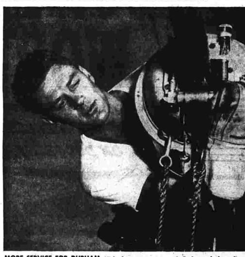
MORE SERVICE FOR DURHAM. High above a country road, Durham telephone lineman James F. Kelly, Jr., starts a cable lashing machine on its way to tie in a section of new cable. Throughout the state, telephone men are using new tools and equipment like this to help speed the construction needed to give Connecticut people the best telephone service in the world.
